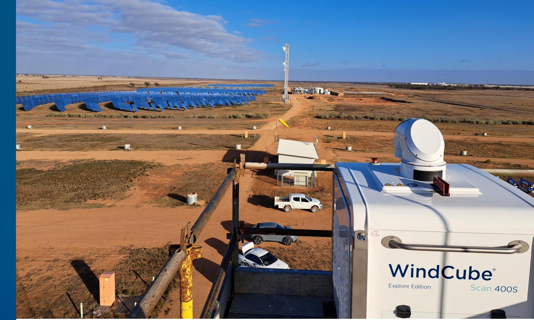
Vaisala WindCube 400S looking over and around the RayGen power plant in Carwarp, Victoria, Australia.
