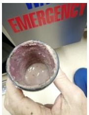
Fig 1. Pink buildup in sink traps
