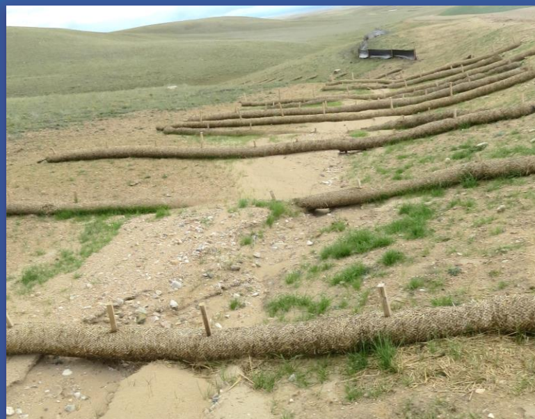
Wattles to prevent sediment run-off
