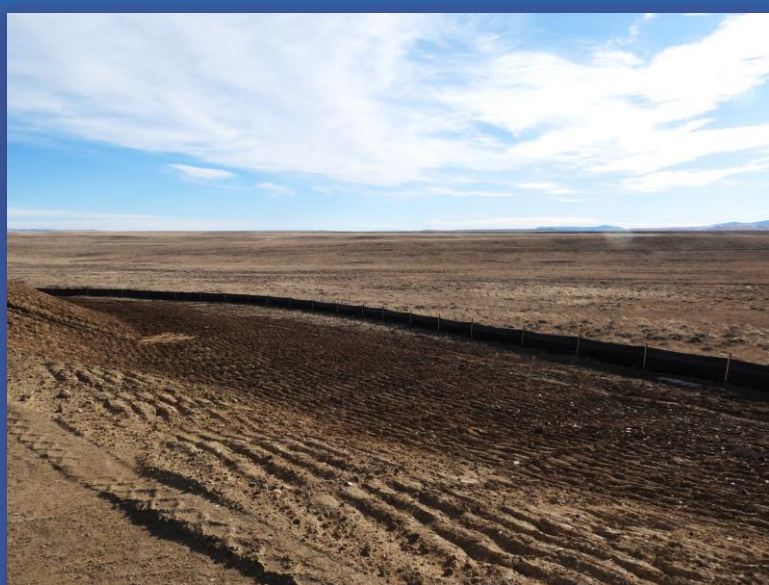
Surface roughening for erosion control
