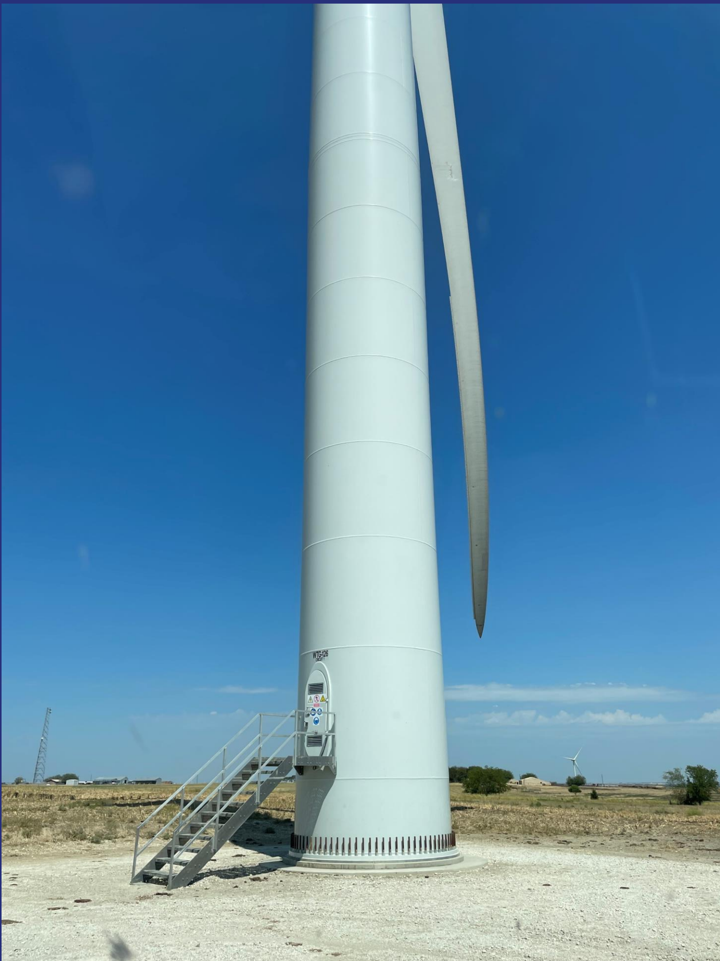
Image depicting the lowest minimum rotor sweep of Model A turbine at the north Texas wind energy facility. The blade tip is approximately 7 m from the ground.
